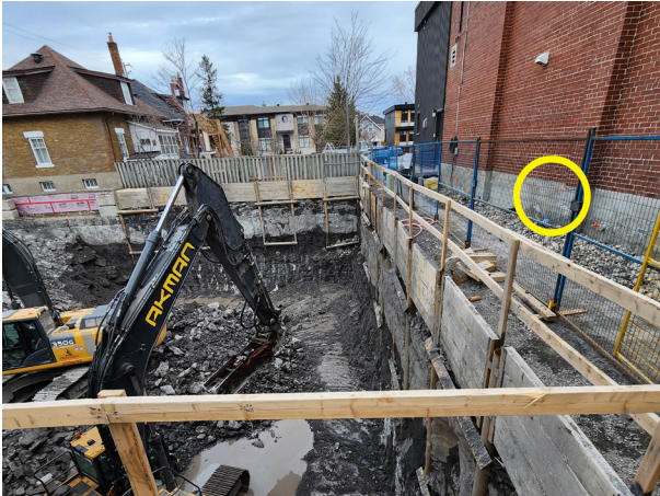
Figure 25. Urban construction site breaking through bedrock.
