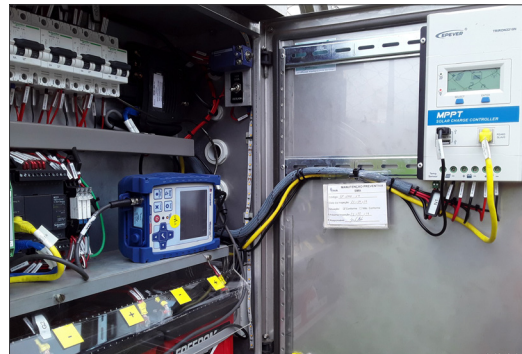
Installed Micromate Monitoring Unit
